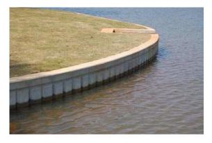
The approximate useful life of a concrete seawall is 40-45 years. The cost can range from \$350 to \$500 per linear foot. We used the lower end of the range for this reserve study. It is advisable to get 3 - 4 bids for seawall work from local and regional contractors. Within our location we would recommend to get bids from Manatee, Sarasota, Pinellas and even more northerly counties.
